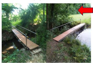
Special thanks to Tony Kaatze assisted by Kevin Reeves as they have refurbished two of our bridges in the last week or so. The lower bridge on Macarthur's and the top bridge at Grubbero have been repaired. They have both been top dressed with 18mm Garnica Duraply which is more waterproof than Marine Ply, it is also very heavy. In addition, they have both had Chicken Wire stapled down for anti-slip.
